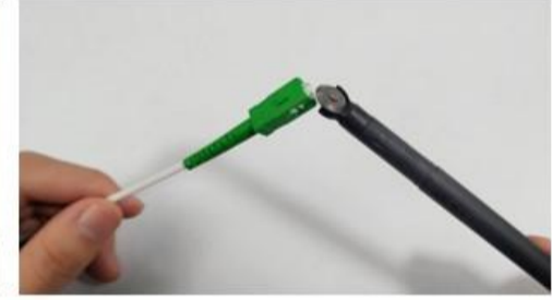
⑨: Use a cutter to remove excess fiber and start polishing
