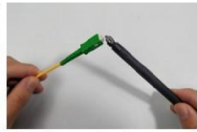
⑩: Use a cutter to remove excess fiber and start polishing
